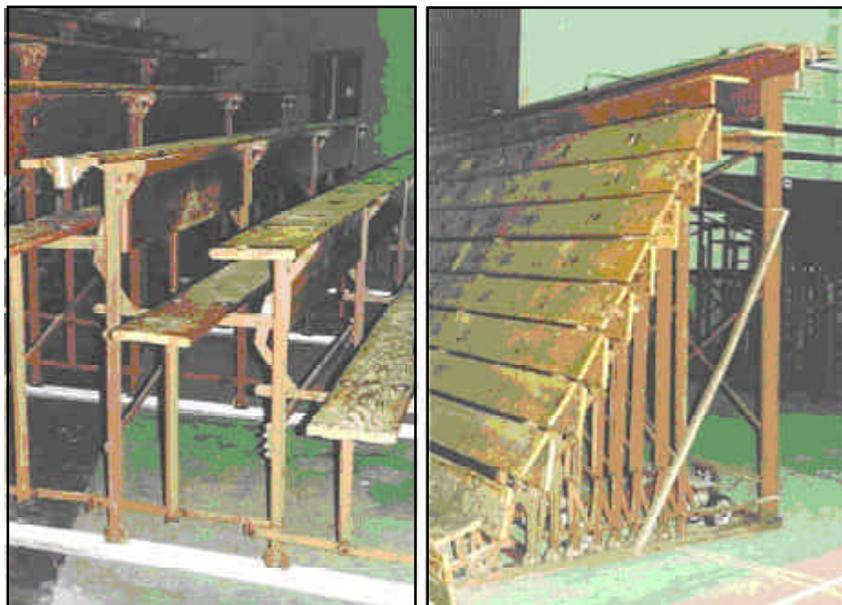
Figure 3: Telescopic bleachers (open and closed positions)
